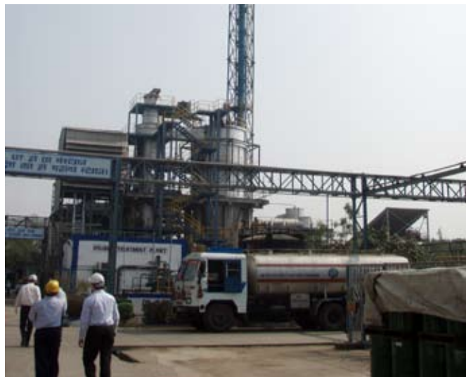
The new incineration plant in India.
