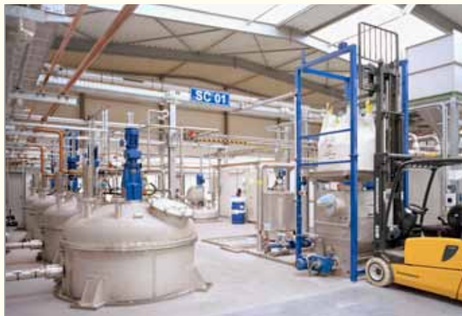
The formulation plant at Stähler in Germany.
