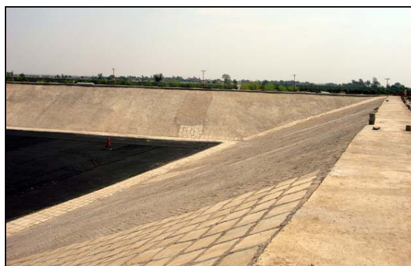
BEIL's depotudvidelse under etablering.
